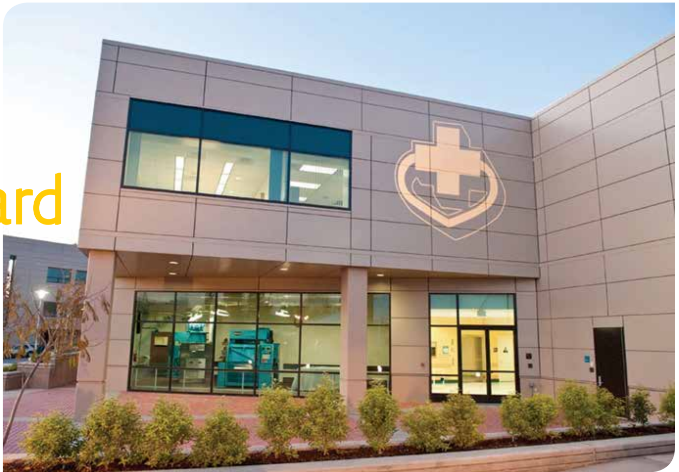
Key elements of the long term Facilities Master Plan including the Central Utility Plant (above) have already been completed.
